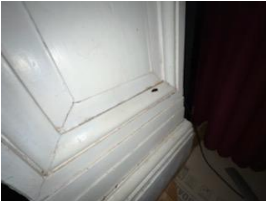
View of white paint on support beam
